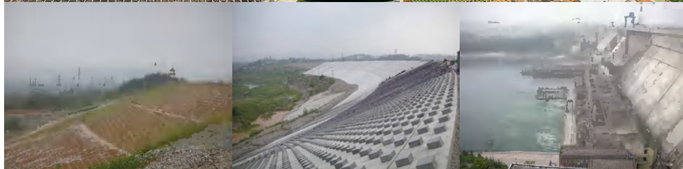
Side of the Danjiangkou Dam
